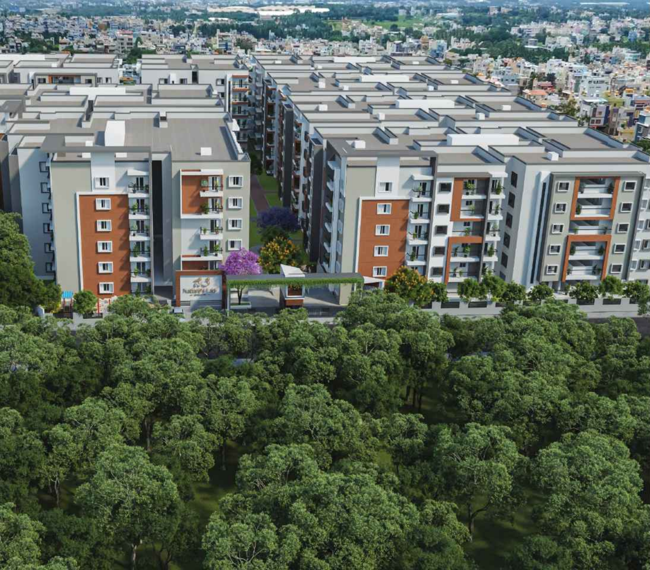
Aerial view of the property and its lush surroundings
