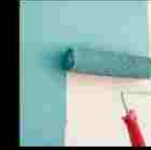
EXTERNAL PAINT WEATHER PROOF TEXTURE PAINT IN BUILDINGS
