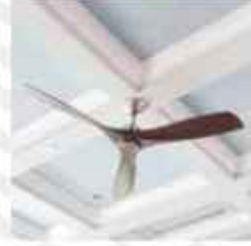
CEILING OIL BOUND DISTEMPER
