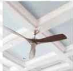
CEILING OIL BOUND DISTEMPER
