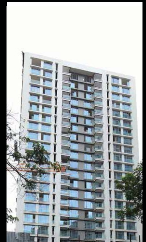
Wing C - Internal painting work in progress
