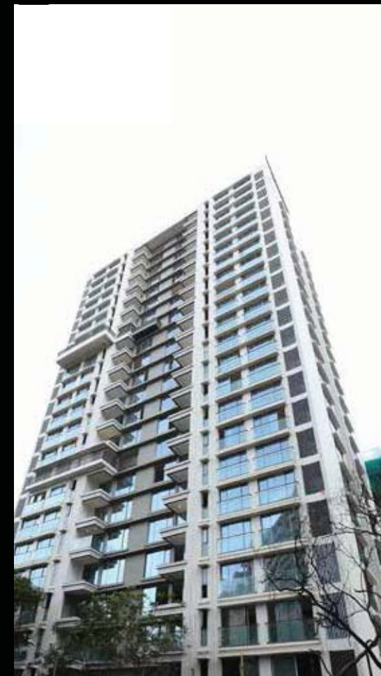
Wing B - Internal painting work in progress
