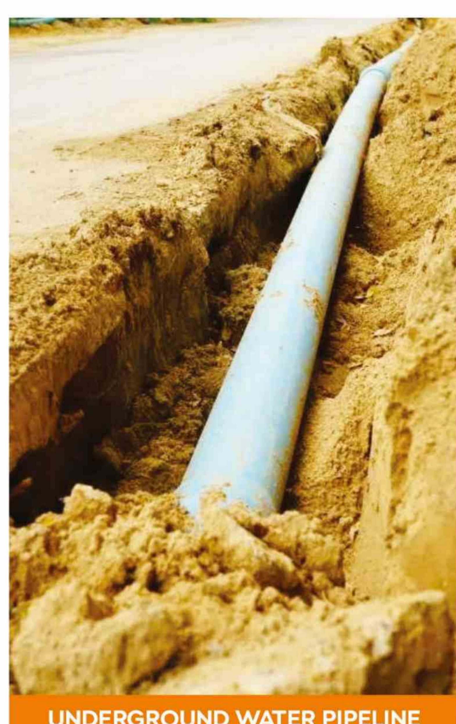
UNDERGROUND WATER PIPELINE
