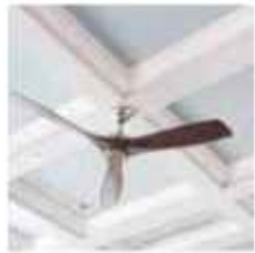
CEILING OIL BOUND DISTEMPER
