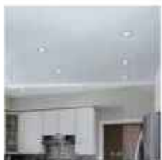
WALL / CEILING OIL BOUND DISTEMPER
