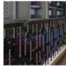
RAILING WROUGHT IRON RAILING
