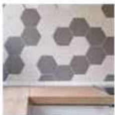
DADO CERAMIC TILES 600 MM ABOVE THE COUNTER
