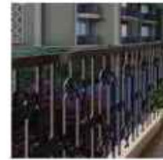
RAILING WROUGHT IRON RAILING
