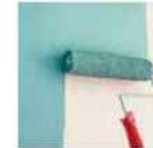
EXTERNAL PAINT WEATHER PROOF TEXTURE PAINT IN BUILDINGS
