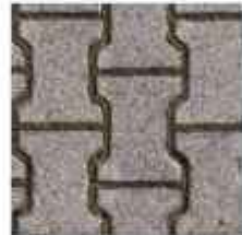
INTERNAL ROADS INTERLOCKING BLOCKS/ TREMIX CONCRETE ROAD
