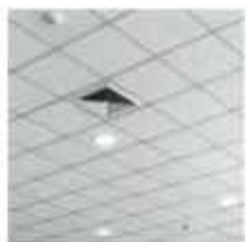
CEILING GRID FALSE CEILING
