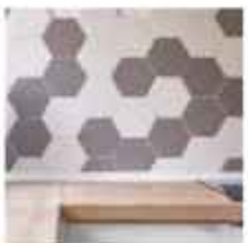
DADO CERAMIC TILES 600MM ABOVE COUNTER
