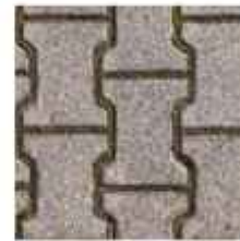
INTERNAL ROADS INTERLOCKING BLOCKS/ TREMIX CONCRETE ROAD
