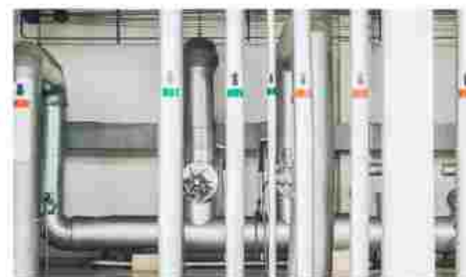
Sewage Treatment System
